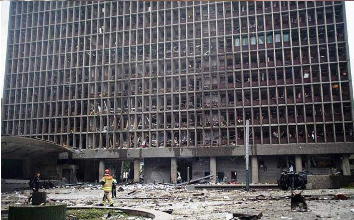
2011. Oslo, Norway. 8 dead, 209 injured. 950 kg ANFO (derived from CAN and diesel and possibly some nitromethane and aluminum).
