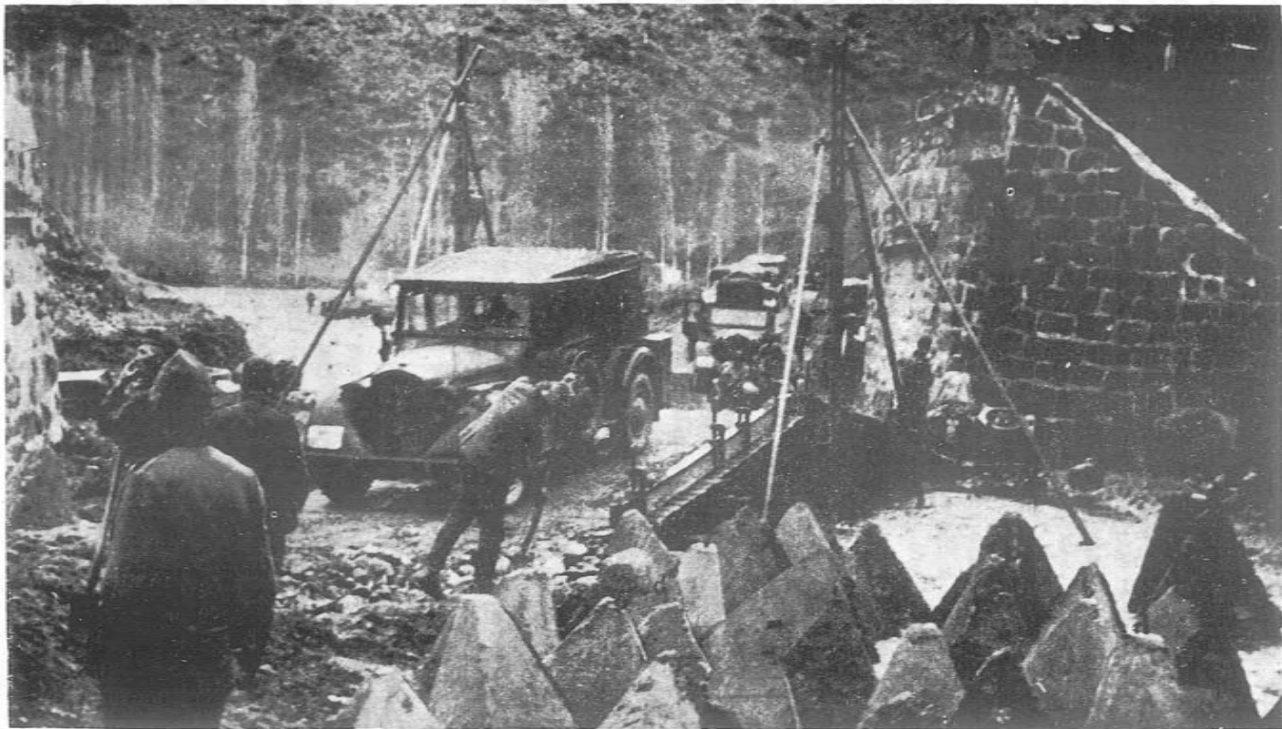
Figure 5. German emergency bridge replaces demolished structure.
